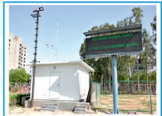
Continuous Ambient Air Quality Monitoring System
